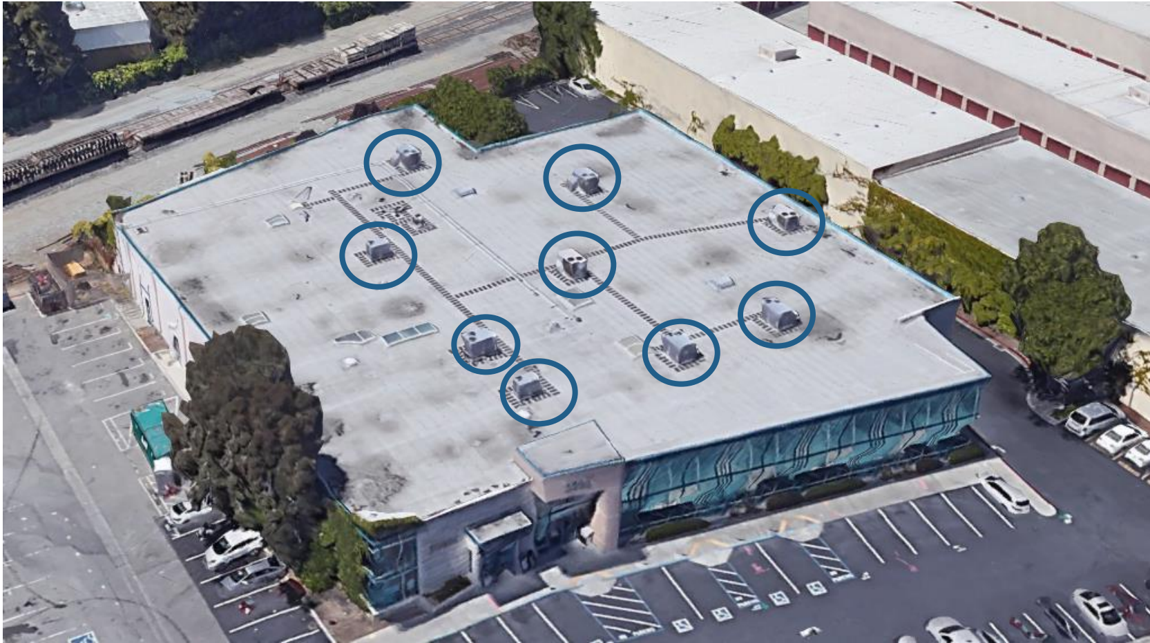
Rooftop Packaged Heat Pumps
